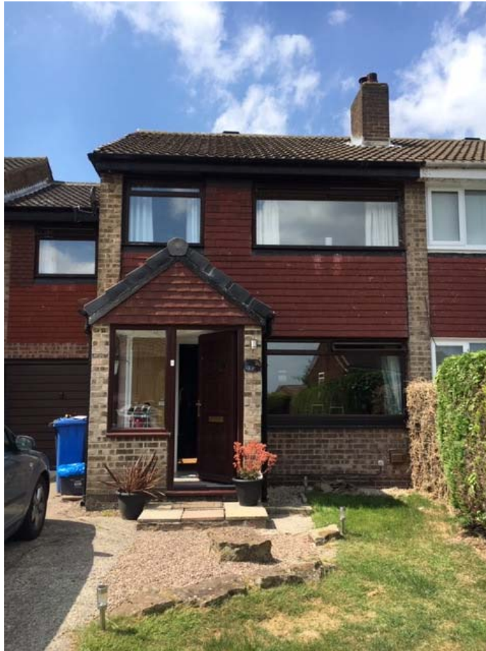
Fig 1: View of existing highway elevation.
